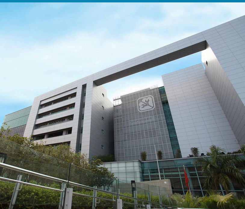
Pilot Scheme on Building-Integrated Photovoltaics (BIPV) at the Electrical and Mechanical Services Department Headquarters
