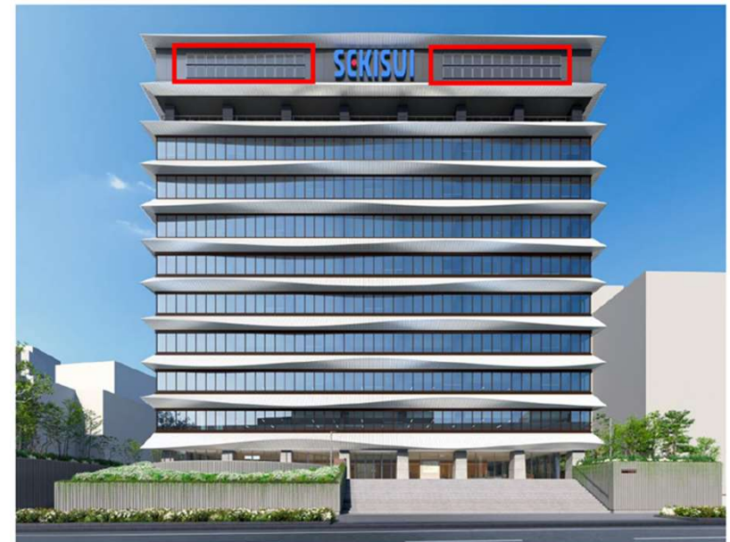
Example of solar panels installed on the walls of buildings
